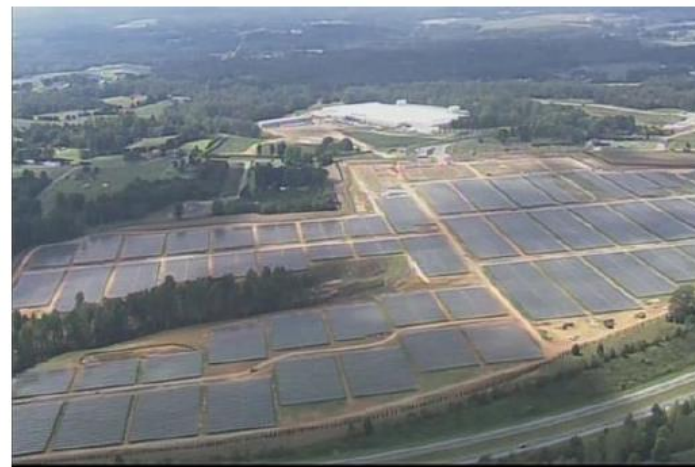
Solar-powered Apple data center
